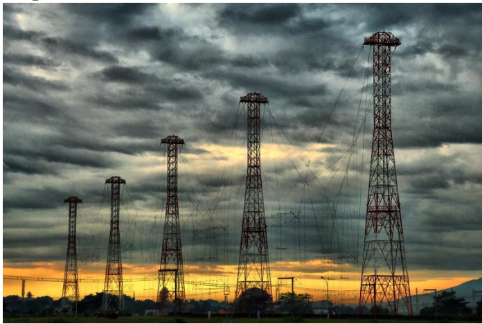
Figure 10: RRI Cimanggis former shortwave towers.
