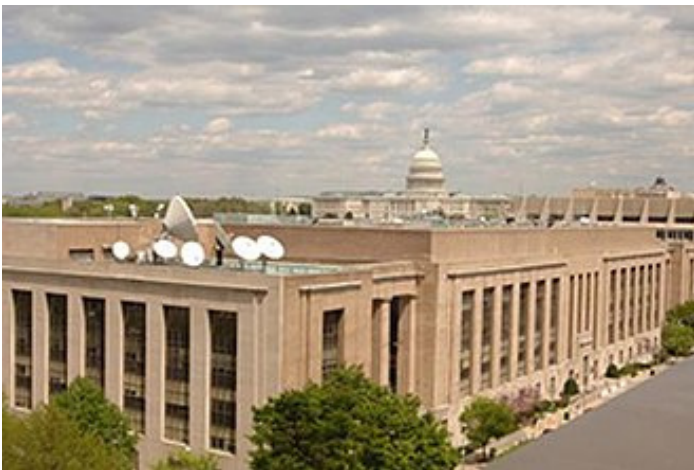
Figure 1: Voice of America's headquarters building in Washington, DC.
