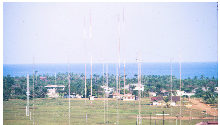
Figure 3: ELWA antenna complex.
