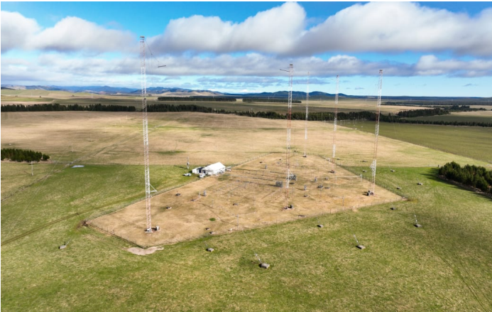
Figure 2: An aerial shot of the new Radio New Zealand transmitter.
