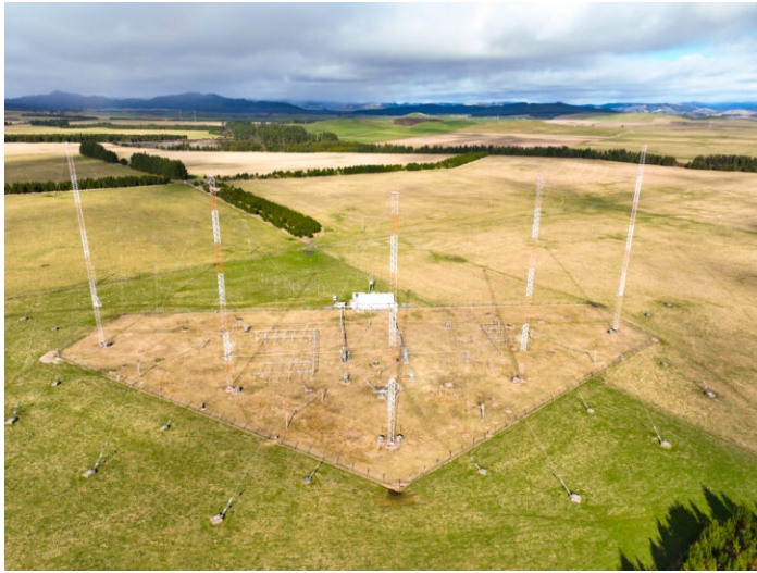
A drone view of the RNZ Pacific shortwave site at Rangitaiki, New Zealand. (Photo courtesy RNZ.)
