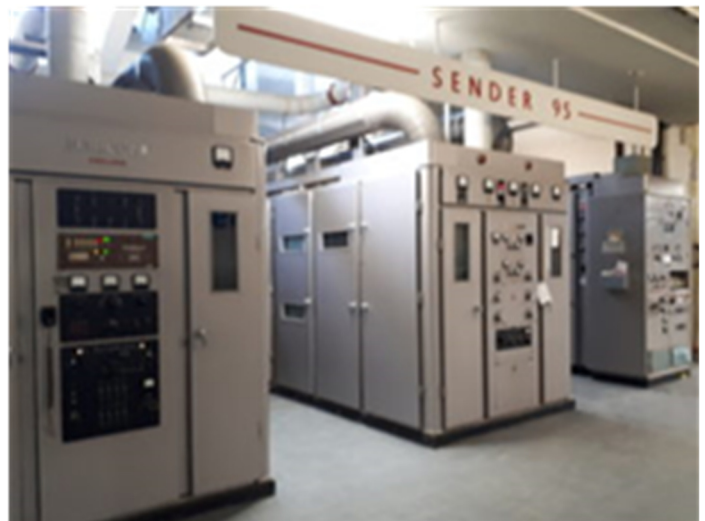
A Marconi BD272 250 kW sender, one the station's oldest transmitters, is still in regular daily use.
