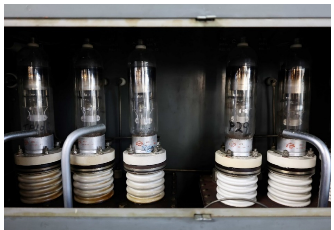
Relic HF transmitter valves at Titahi Bay (Photo courtesy Radio New Zealand)
