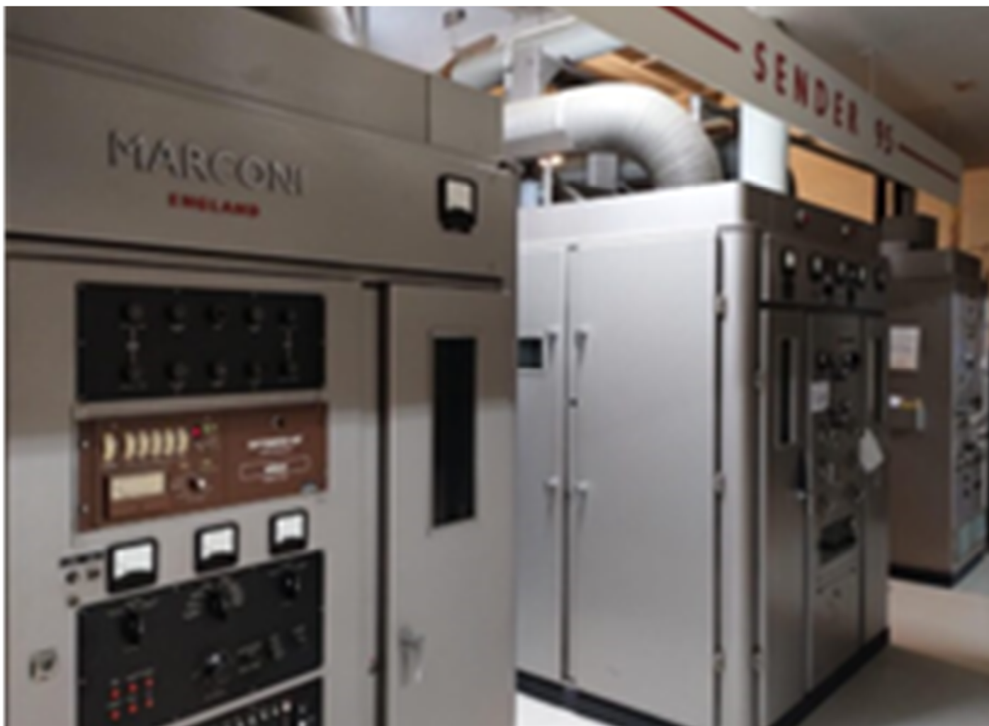
This Marconi BD272 transmitter was installed in 1963 and remains in working condition; it is the oldest at the site.
