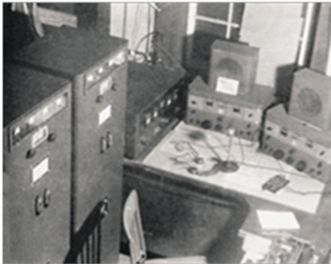
US Weather Bureau radio station on Swan Island. The two tall cabinets on the left house the Navy's CW transmitters, with the 100-watt transmitter for the 14 MHz band (HT9) in the next corner. On the table are two AR-77 receivers as well as headphones, a microphone and a Morse key (1940). Photo: Steve Paull
