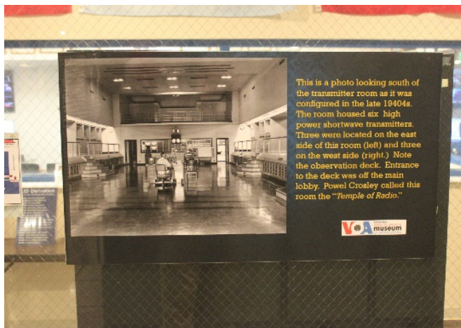
Photo of Transmitter Room
