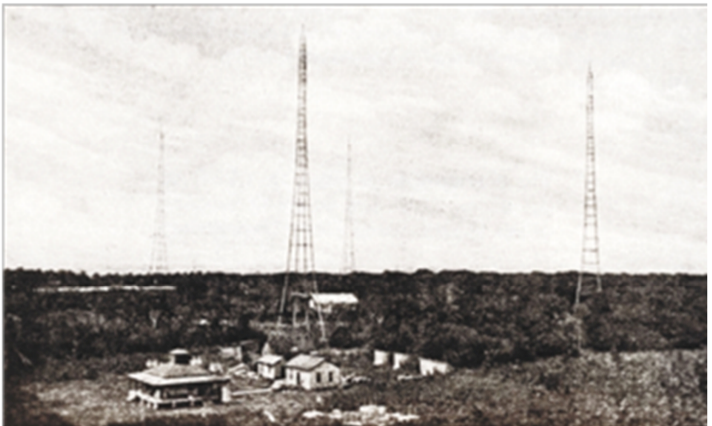
The antenna system on Swan Island, which was expanded around 1913. Photo: WSA.
