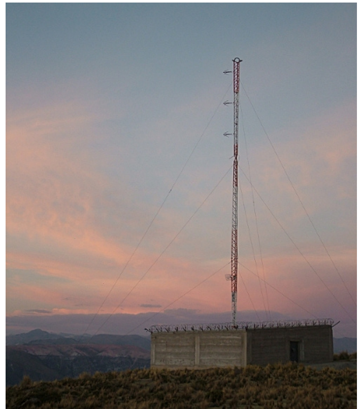
Radio Senda Cristiana transmission site with FM antenna.
