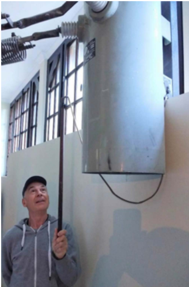
Dave Kenny with balun transformer at Encamp
