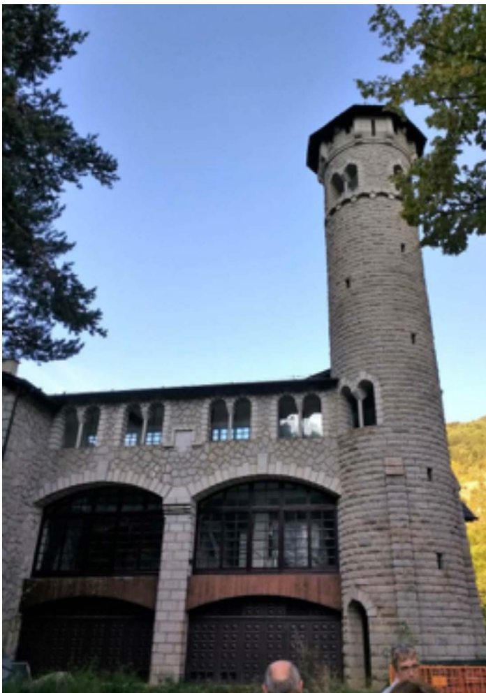
Turret on Radio Andorra transmitter building.
