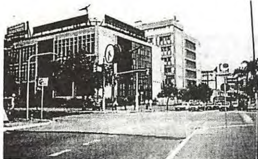
Fig 4: Radio Gaúcha is located in a modern building in Ipiranga Avenue, a short distance from downtown.
