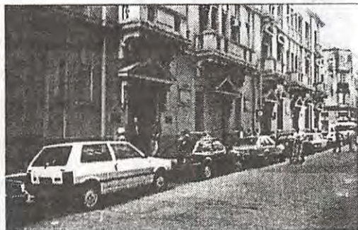
Fig 3: Rádio Guaíba is located in an old but well preserved building in Caldas Junior st., a narrow street in the old downtown.
