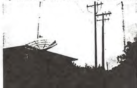
KWHR Satellite Dish and Antenna
