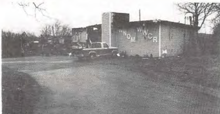
The walls on the right side of the building remained standing.
