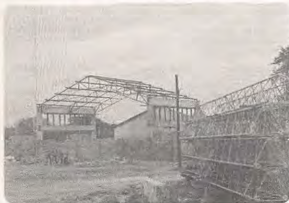
VIEWS OF THE SITE WITH ANTENNAS ON THE FOREGROUND
