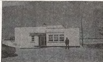
CHU transmitter building with Hamilton in front.
