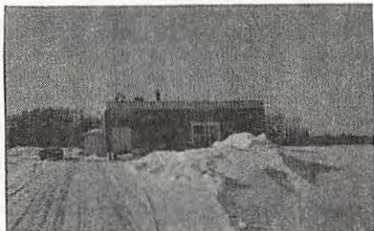
Stanley Corners Monitoring Station from the driveway.
