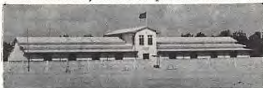
***RADIO MALDIVES BUILDING***
