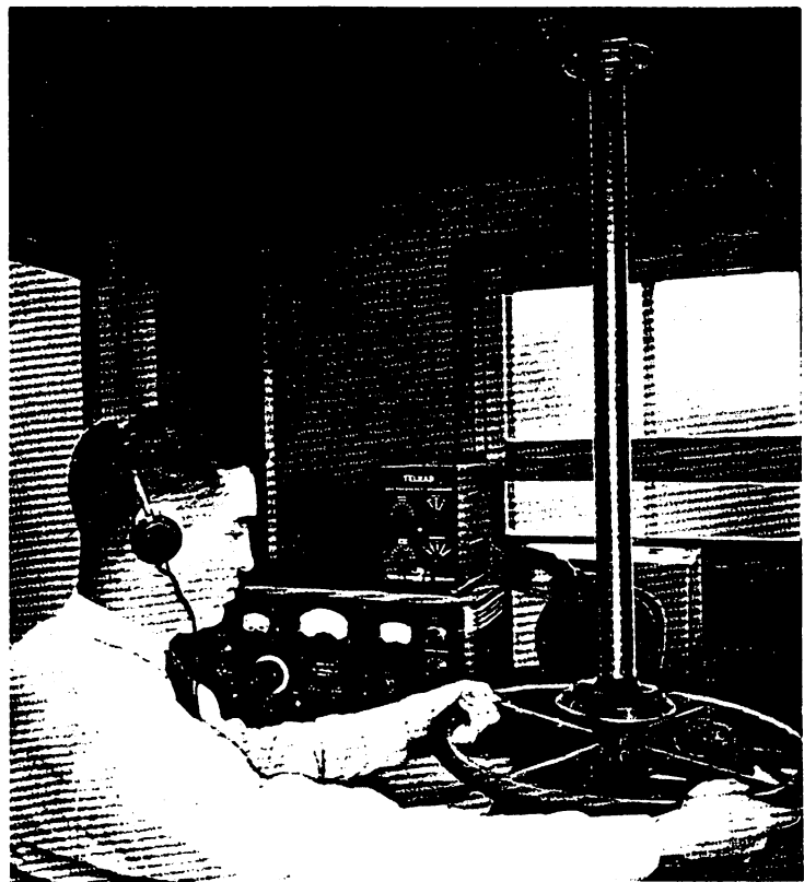
FIGURE 11. Adcock Array DFing Hut
