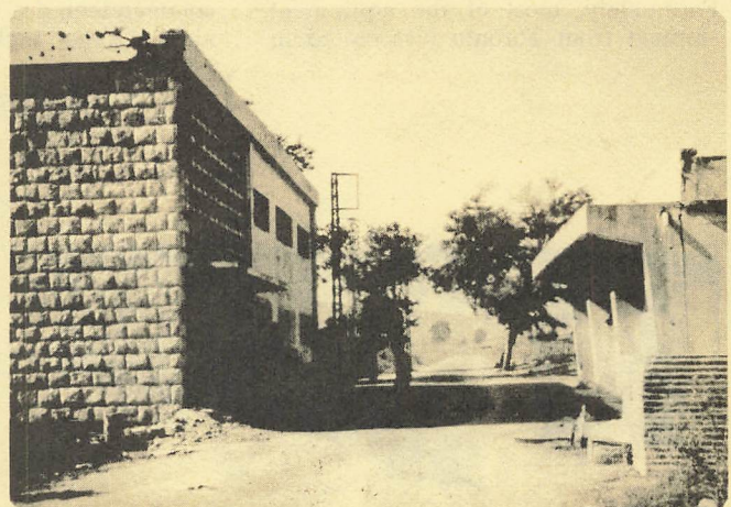
Building at left was renovated for studios of Free Lebanon's "Voice of Hope".
